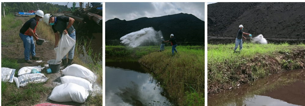
Kegiatan water treatment settling pond MCT 1 dan settling pond MCT 2
